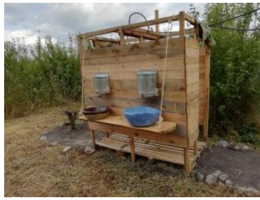
Compost toilette made with cob. Solar showers.
