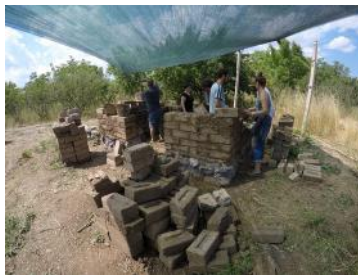
Preparation of Cob and building made with adobe bricks.
