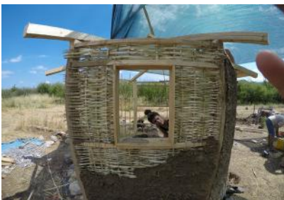
During a workshop we build a little house with wattle and daub and a reciprocal roof.
