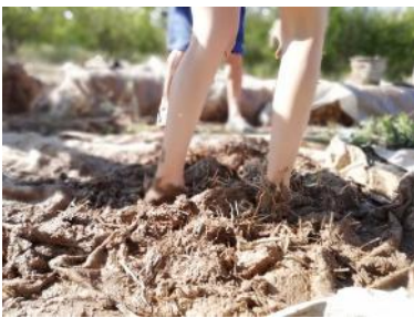
Preparation of Cob and building made with adobe bricks.
