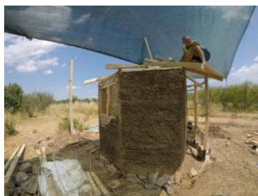
During a workshop we build a little house with wattle and daub and a reciprocal roof.
