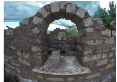
Preparation of Cob and building made with adobe bricks.
