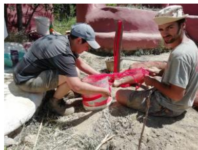
Earthworks for a natural pool
