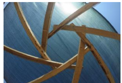
During a workshop we build a little house with wattle and daub and a reciprocal roof.
