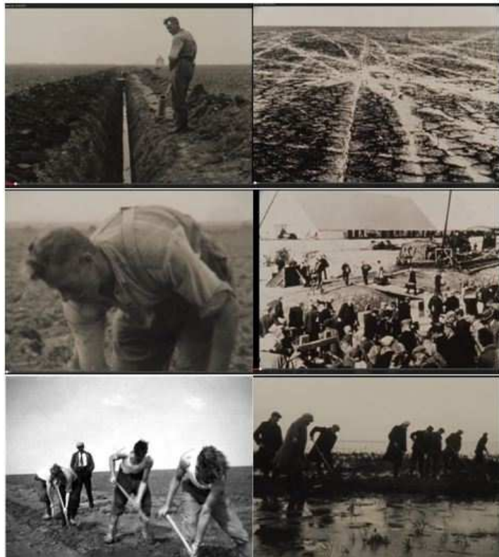
Figure 1 Creating the drainage system in the polder by hand.
